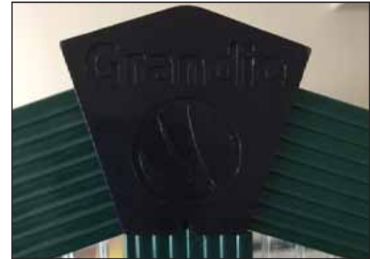
Exterior view of mid roof cap JG01.
